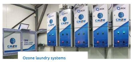
Ozone generator integration to the dosing system for environmentally friendly cost-effective ozone washes that reduce hot water consumption.
